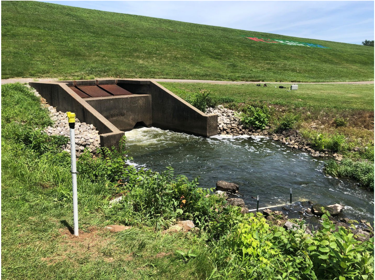
Figure 40. The pressure transducer at West Boggs Lake Outflow. The pressure transducer was used to measure discharge or the amount of water leaving the lake. Once discharge is measured a water budget for a lake can be created.
